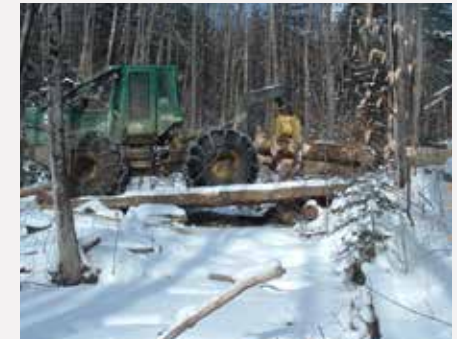
Temporary Skidder Bridge
