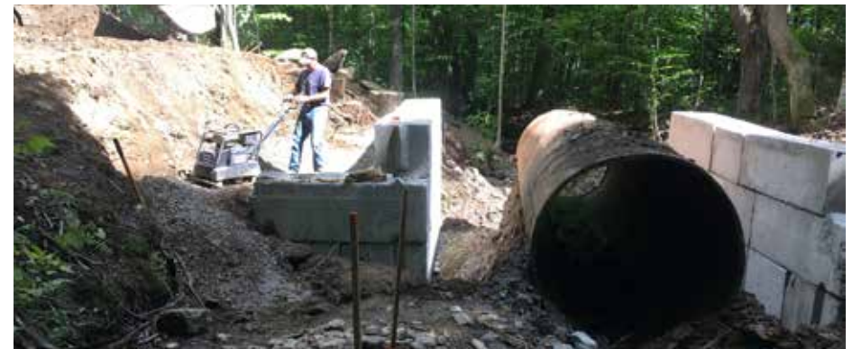
Replacement of an undersized culvert with bridge.
