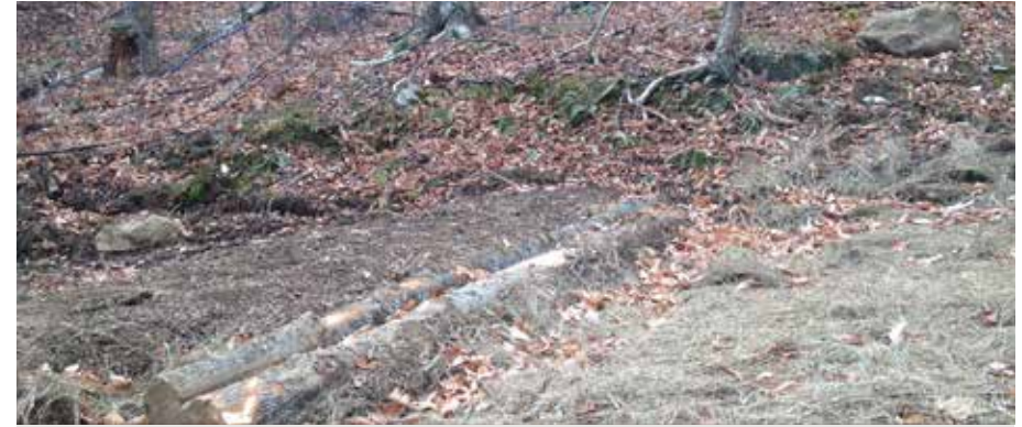
Log-reinforced water bar
