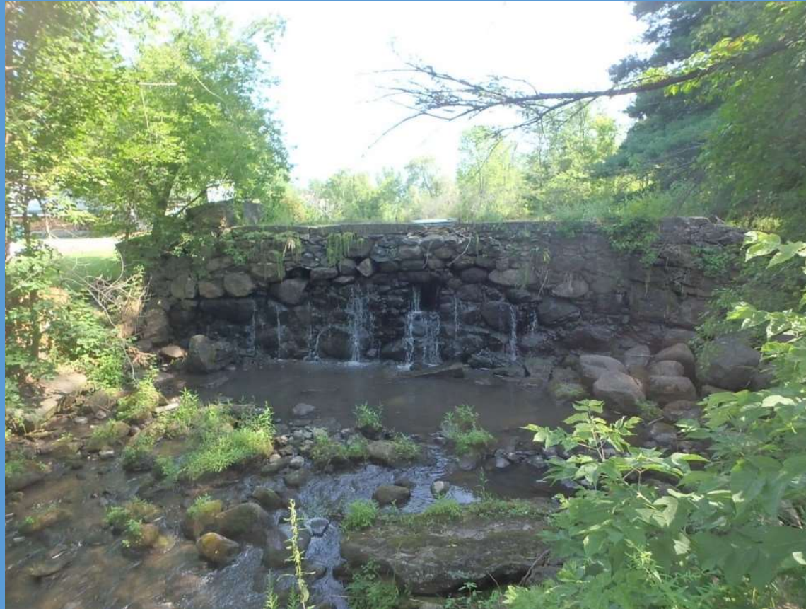
Looking Upstream at Old Stone Dam 2017
