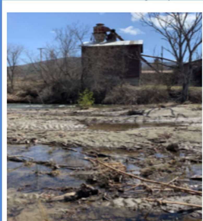
Flood damage after Tropical Storm Irene
