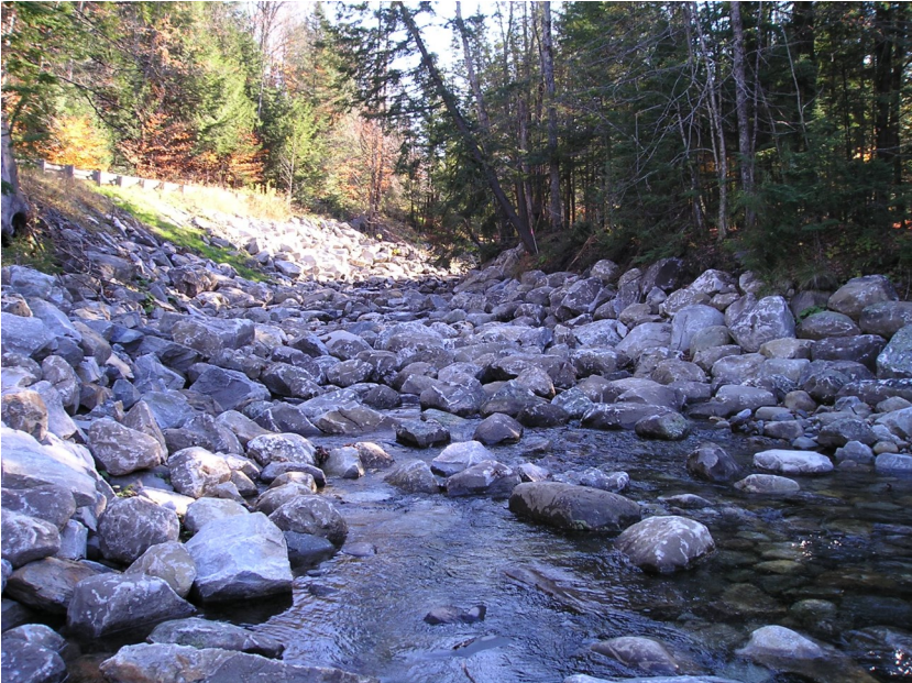
Figure 3. Bed armor creates an immobile surface to protect the underlying bed from eroding downward.
