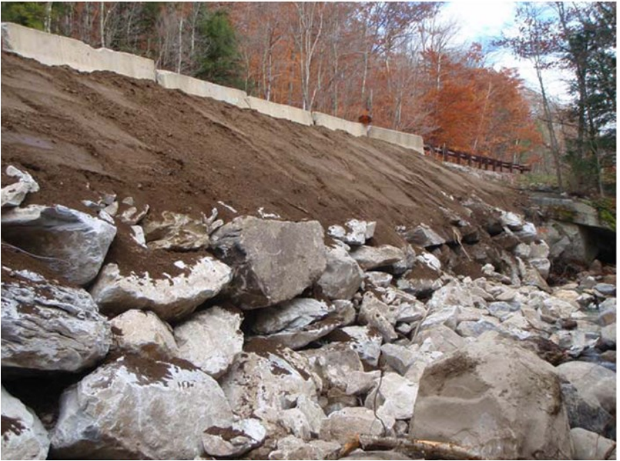
Figure 2. A placed Rip Rap Wall creates lateral channel stability. The steep slope at toe results in less horizontal fill which allows for attainment of full bankfull channel width in confined settings.
