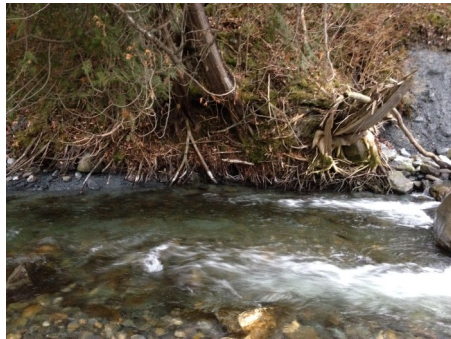
Example of freshly exposed roots as a head-cut moves upstream
