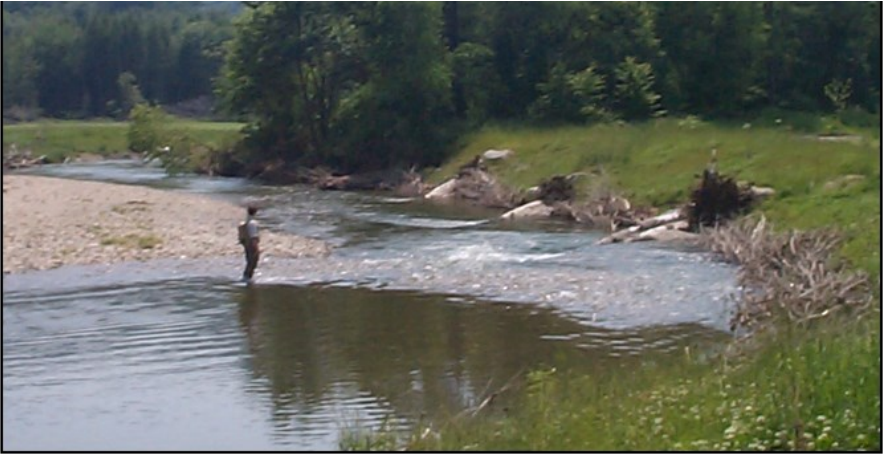
Figure 6. Log J-hook vanes meet the same objectives as the rock J-hook vanes but can be more difficult to construct and have a shorter life expectancy. However, in situations where large rock is unavailable they can be a viable alternative to the rock J-hook vane.
