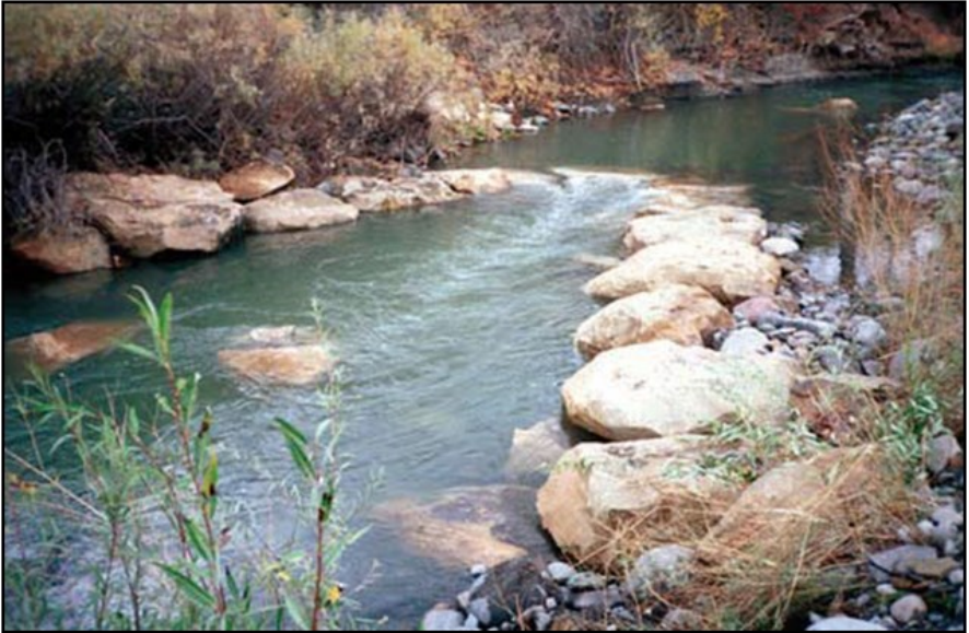
Figure 4. Rock cross-vanes (looking upstream) meet multiple objectives including bed and bank stabilization and sediment transport by creating a stable point in the channel that dissipates and redirects erosive energy as well as habitat by providing deep pools.
