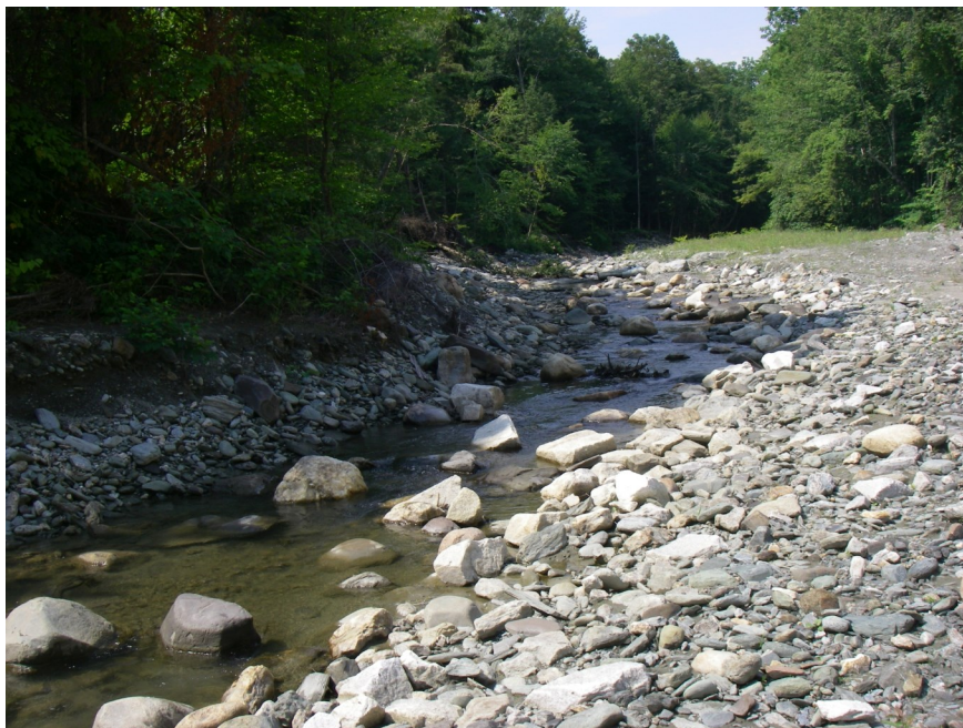
Figure 7. Random boulder placement meets multiple objectives including channel stability and habitat maintenance by creating roughness that dissipates erosive energy in a way that results in the creation of small scour pools.
