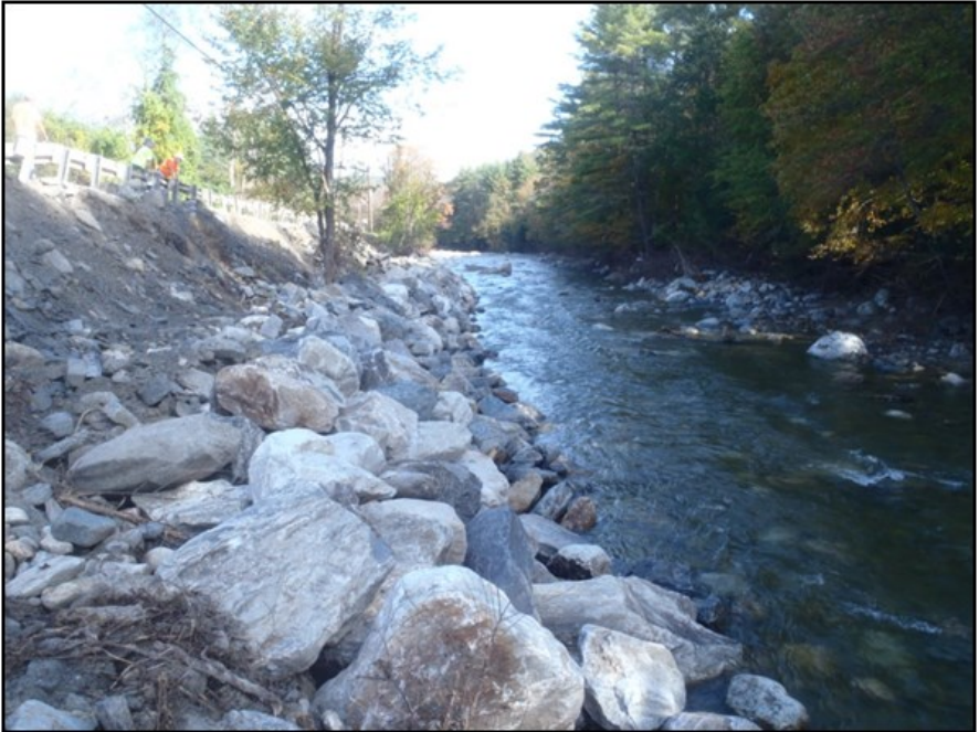
Figure 1. Stone Fill serves as an immobile surface that protects the underlying bank from erosion.
