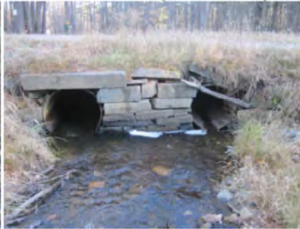
US CULVERT (FACING DS):
