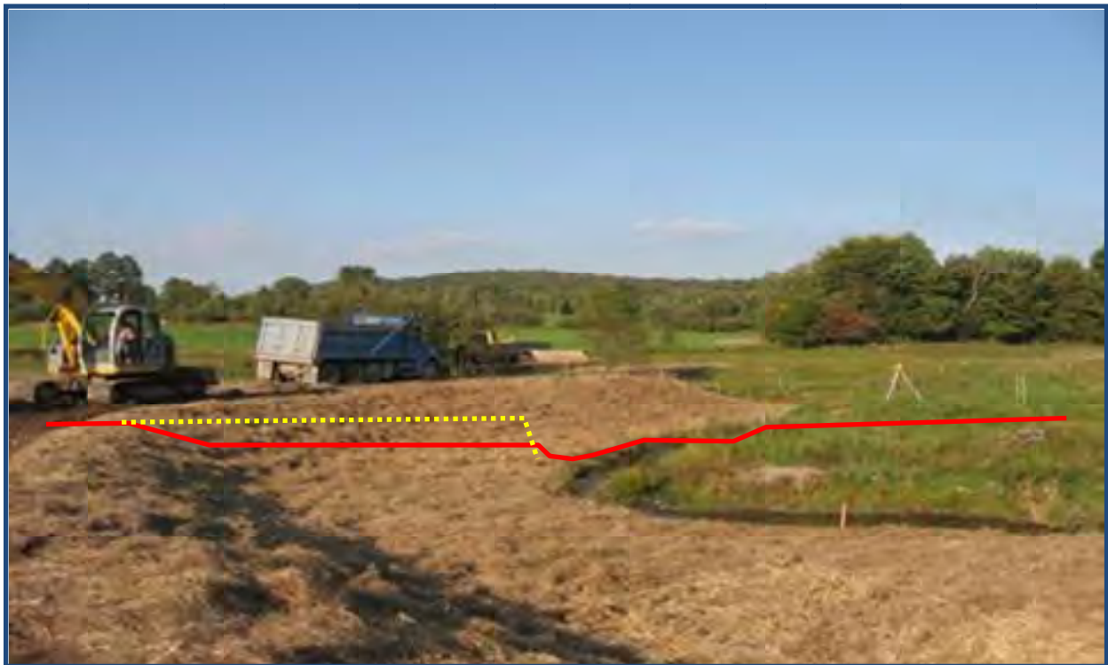
Figure 5.6-3: Floodplain restoration along Wanzer Brook in Fairfield, Vermont by lowering the elevation of the floodplain (between the dotted and solid line). (Source: S. Jaquith, VTANR)
