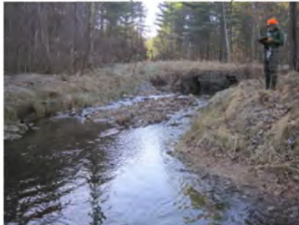
DS CHANNEL (FACING US):
