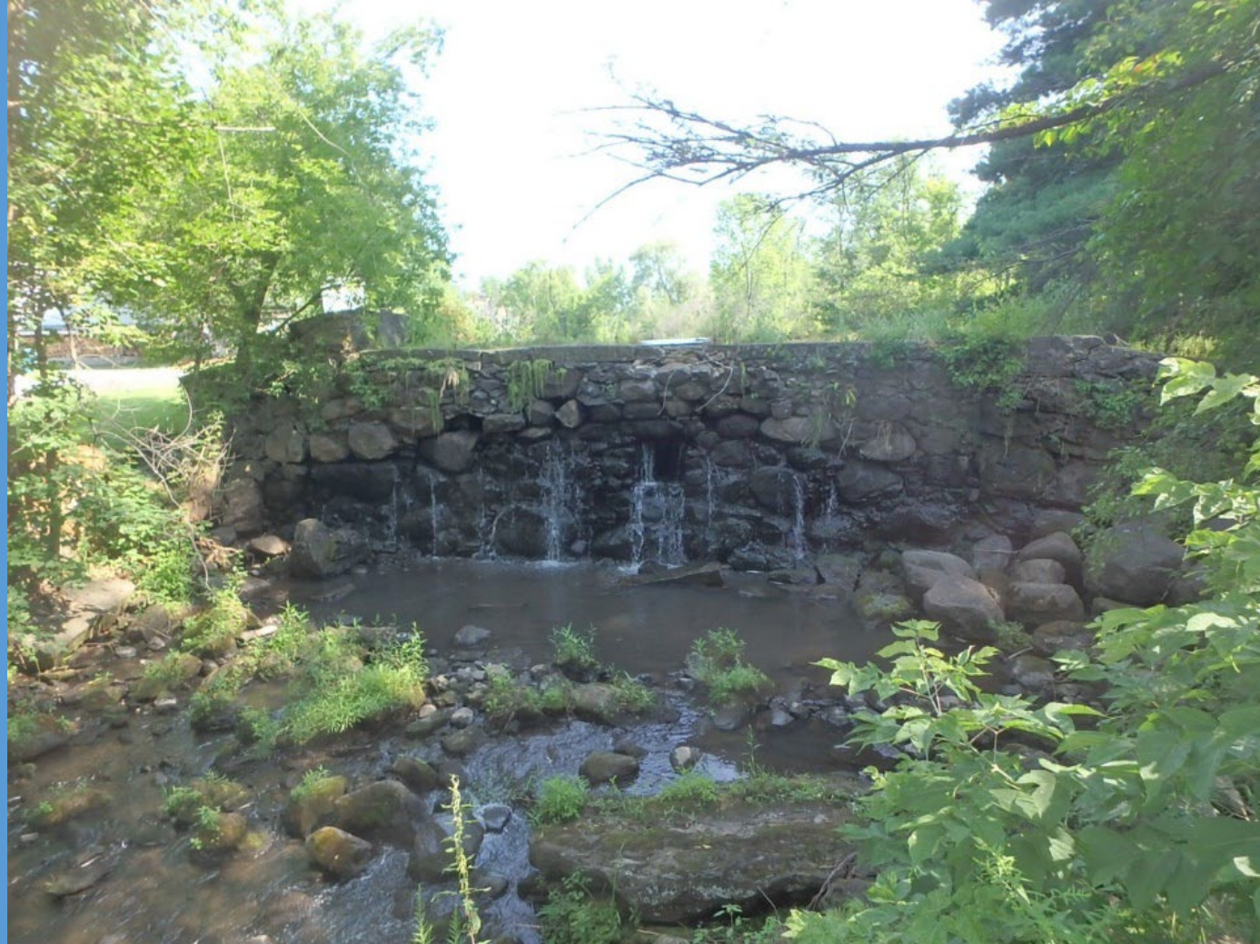
Looking Upstream at Old Stone Dam 2017
