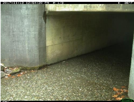
Figure 24. Examples of old box culverts with “sheetflow concrete” movement surface. Site 30-22 (West Townshend) and 15-76 (Cambridge, Marangelo and Farrelll 2016).
