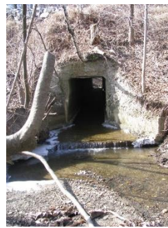
Figure 24. Examples of old box culverts with “sheetflow concrete” movement surface. Site 30-22 (West Townshend) and 15-76 (Cambridge, Marangelo and Farrelll 2016).
