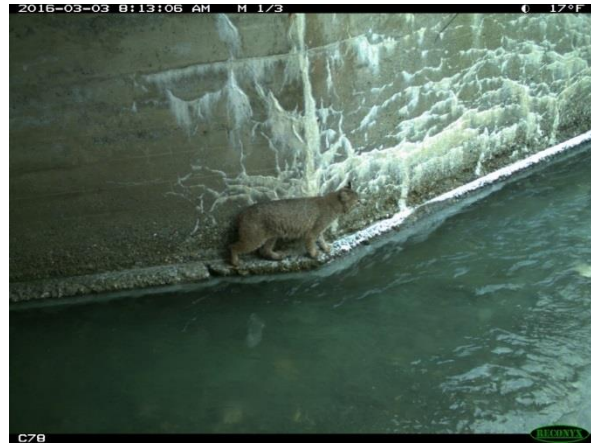
Figure 23. Bobcat through passages at span with footing shelves structure design types (Site 114-20 (left) and 4a-13 (right)).
