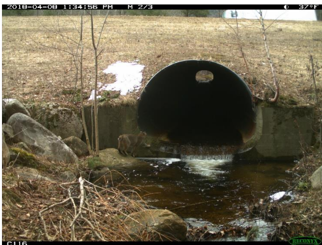
Bobcat at squash pipe 7-19-5, Sunderland
