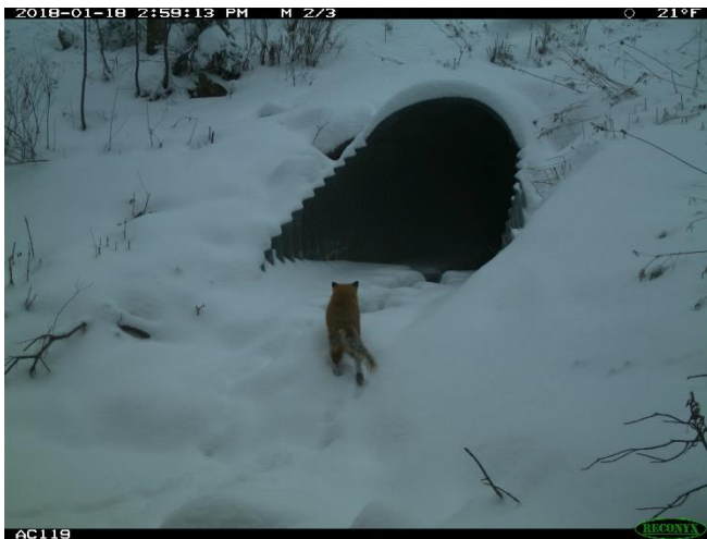
Fox approaching pipe culvert 9-17, Woodford (did not enter)
