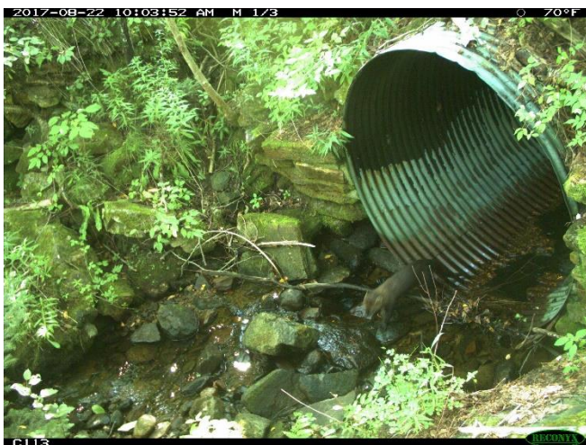
Fisher at pipe culvert 155-6, Mt Holly
