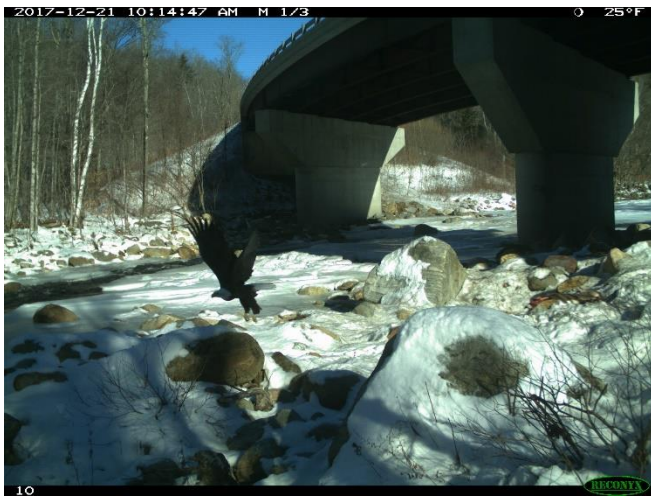
Bald eagle at span 9-25b, Searsburg
