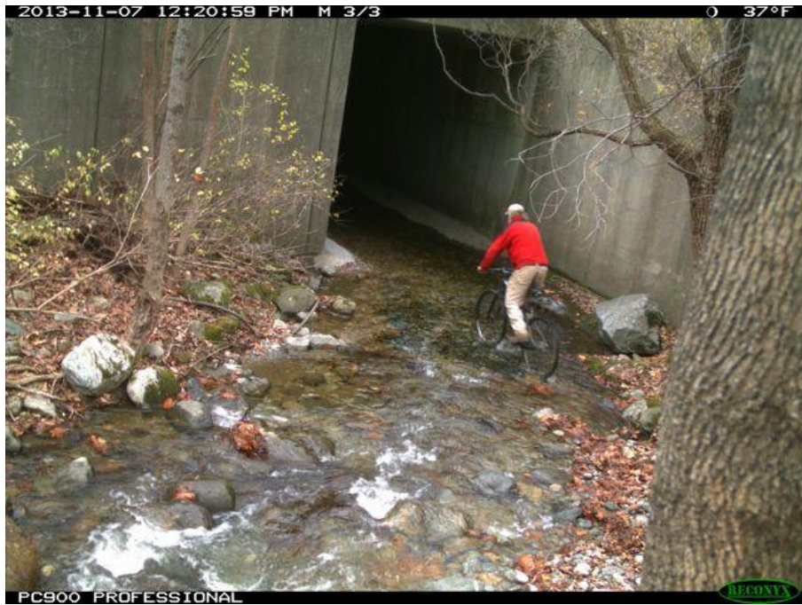
Pineo Brook inlet, north side of US Route 2, facing south
