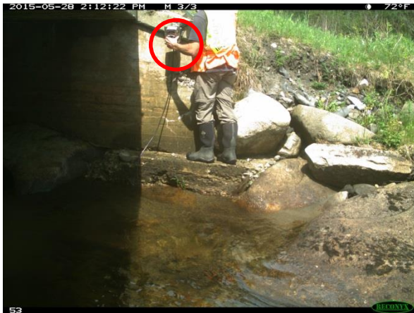
Downstream left descending abutment, camera
