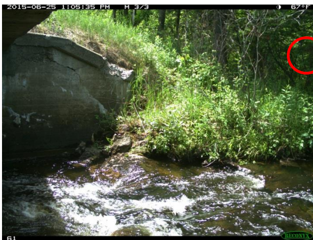
Upstream right descending abutment, camera
