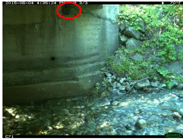
Upstream right descending abutment and camera
