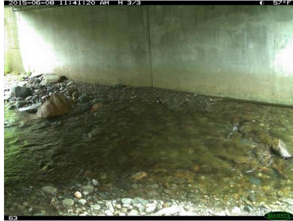
Right descending abutment
