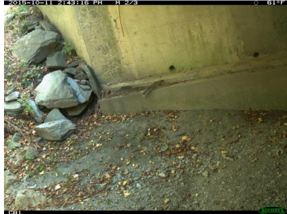
Upstream left descending abutment
