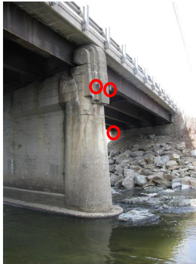
Bridge pier and right descending bank cameras
