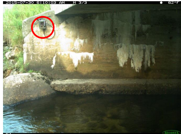
Downstream right descending abutment, camera
