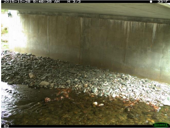
Left descending abutment
