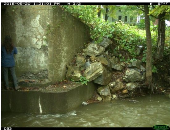
Upstream right descending abutment
