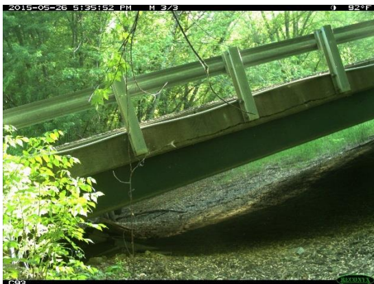
Downstream, right descending bank abutment
