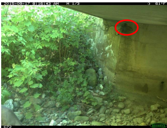
Downstream right descending abutment and camera
