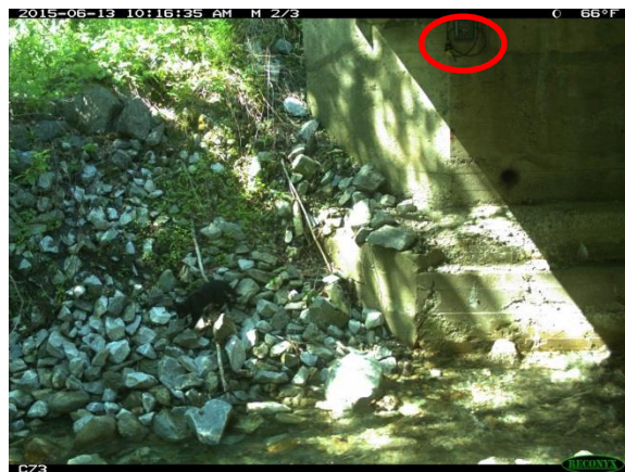
Upstream left descending abutment and camera
