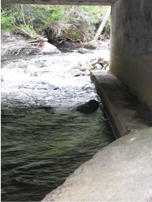
Figure 7. Concrete “abutment shelf” at Site 114-20 in Newark
