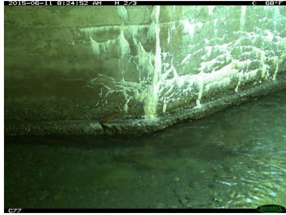
Upstream left descending abutment
