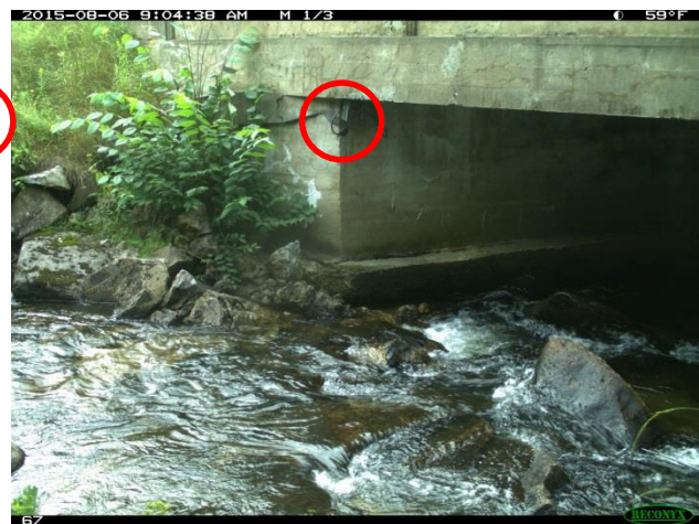
Upstream left descending abutment, camera
