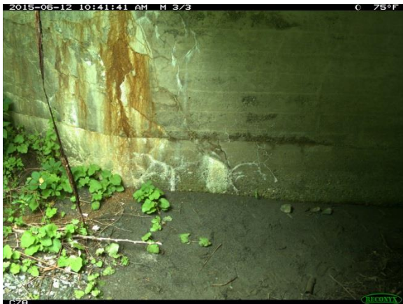
Downstream right descending abutment
