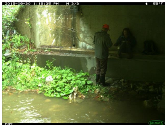
Downstream right descending abutment
