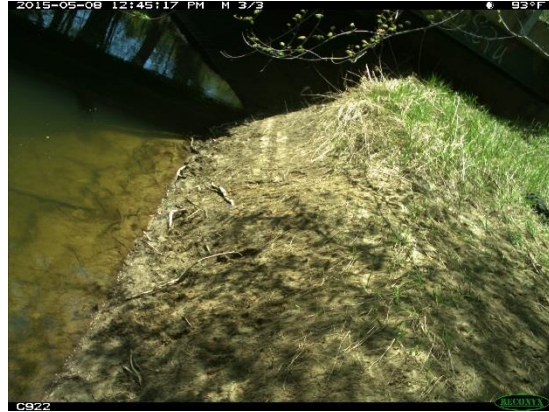
Downstream, left descending bank
