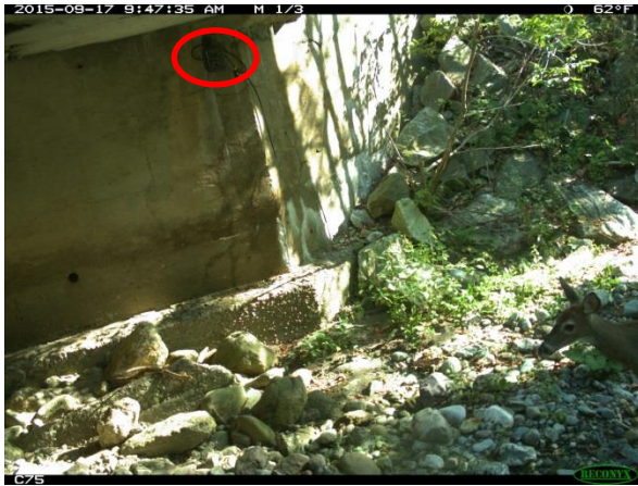
Downstream left descending abutment and camera
