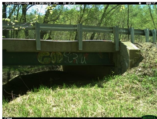
Upstream, right descending bank abutment
