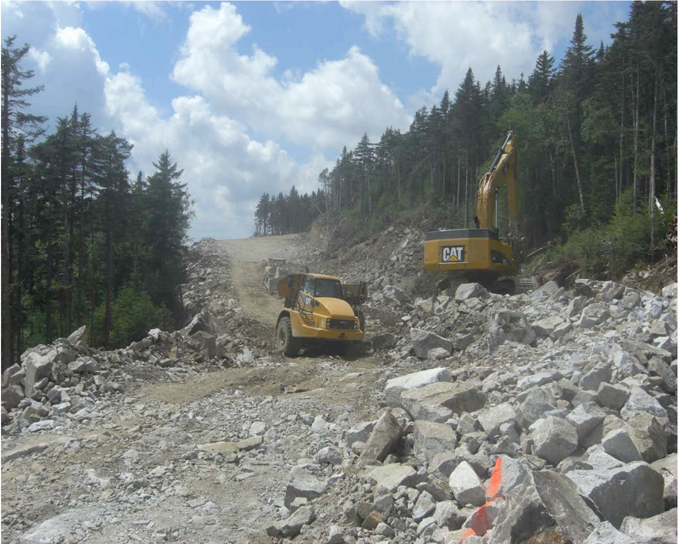
Road to Mt. Kelsey After Blasting
