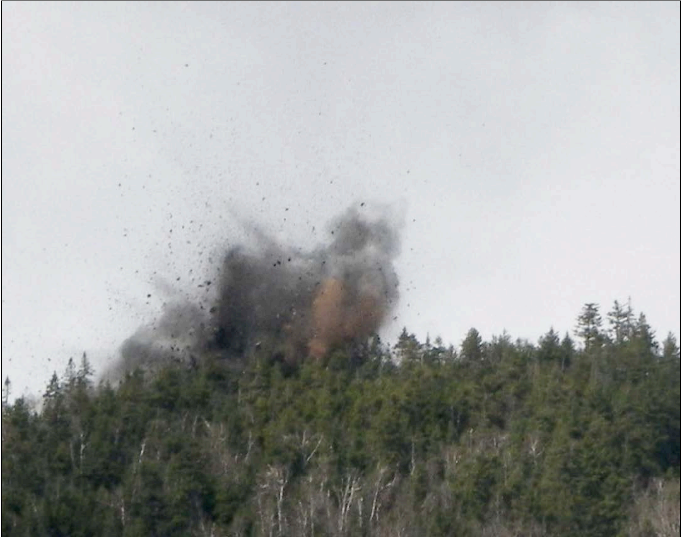
Uncontrolled Blasting, Lowell Mountain, Vermont
